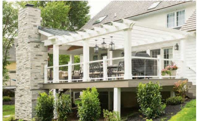
18' x 18' Somerset 8" Square Columns, Electrical.
